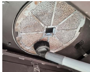
Cleaning of catalytic converters using a vacuum cleaner with brush attachment
